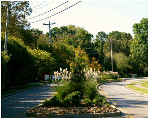
Suburban streets can have medians (above) as a method of access management, and to create a consistent community character.
