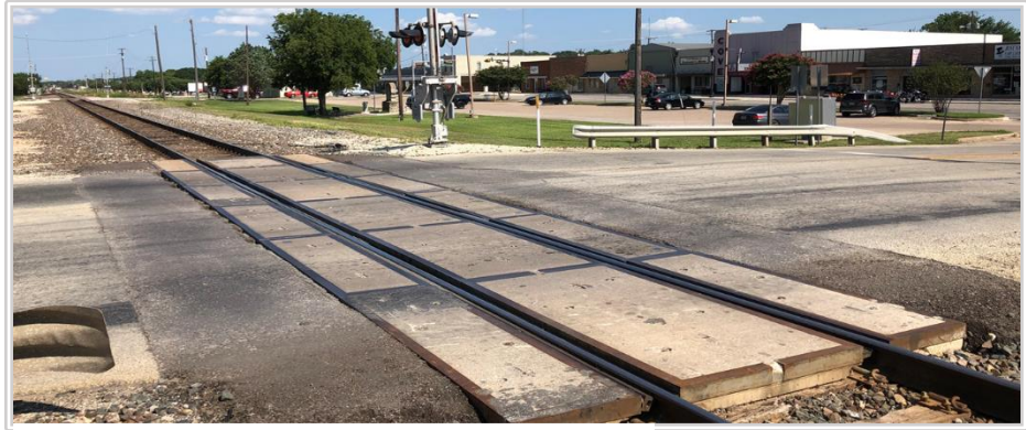
At Grade Railroad Crossing at 1 st Street
