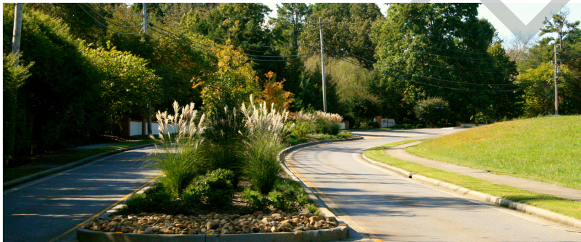
Suburban streets may have medians (above) as a method of access management, and to create a consistent community character.
