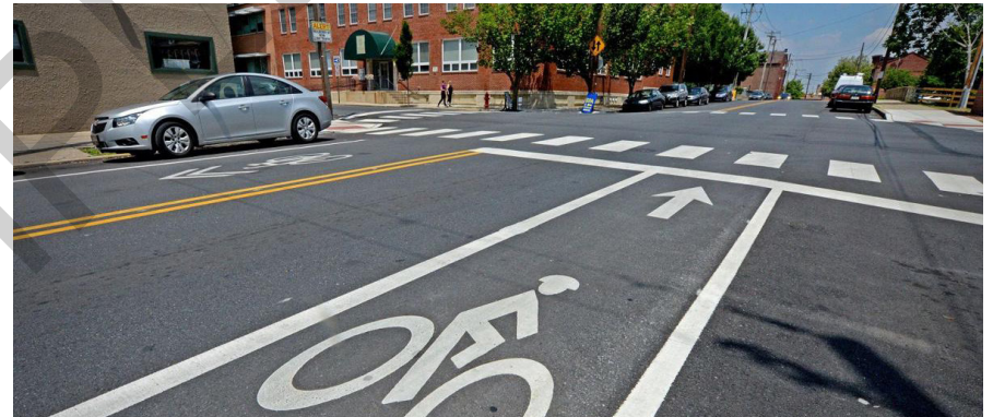
Urban streets can be candidates for lane reductions. The street above was converted from a four-lane minor arterial street into a three-lane avenue with on-street parking, bicycle lanes, and intermittent medians (above).
