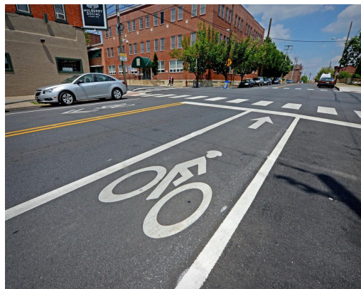
Urban streets can be candidates for lane reductions. The street above was converted from a four-lane minor arterial street to a three-lane avenue with on-street parking, bicycle lanes, and intermittent medians (above).
